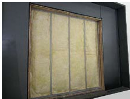
1 #1050R Self-Adhesive Tape, applied to the studs
