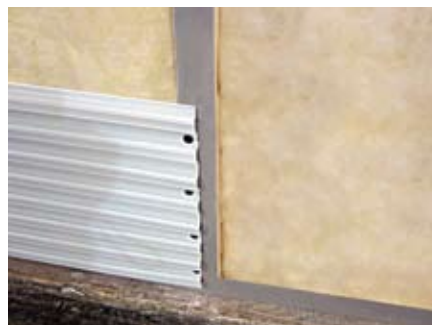
2 #1033 - Primary Insulator, fastened horizontally to the studs
